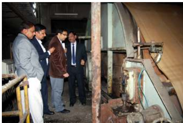
Members of PRC viz Shri M. Salahuddin, MoEF Shri A.K. Vidyarthi & Dr. S. Panwar, inspecting the Lignin Precipitation System installed by Kuantum Papers under the Project
